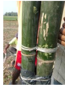
Floor post and roof post connection
