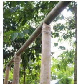
Roof beam and post connection
