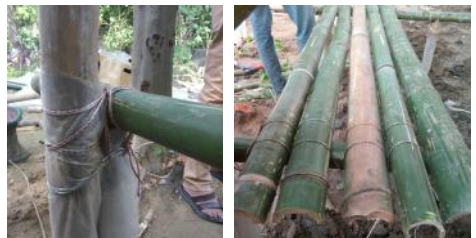
Picture 2 : Floor post, beam and joist connection
