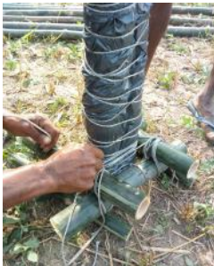
Post and anchorage connection
