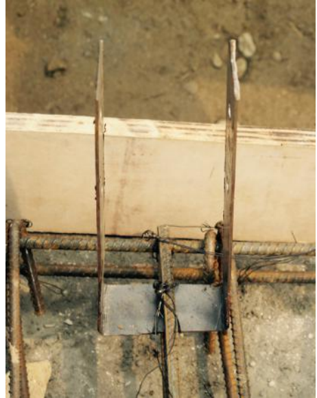
Picture: Connection between reinforcing steel and U-straps
