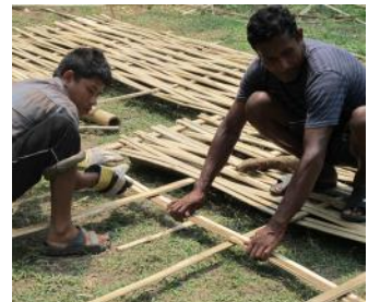
Walls built aside on ground
