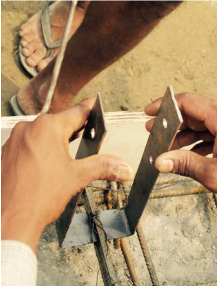
Picture: Connection between reinforcing steel and U-straps
