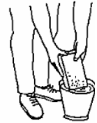
Wet the bricks before laying them
