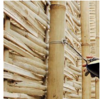
Walls attached to structure on outside using wires/nails
