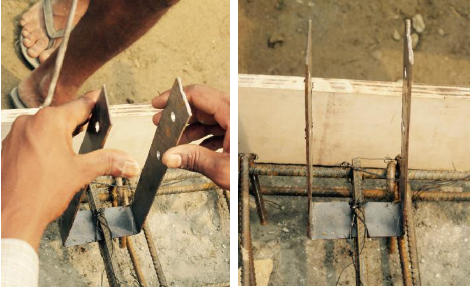
Picture: Connection between reinforcing steel and U-straps
